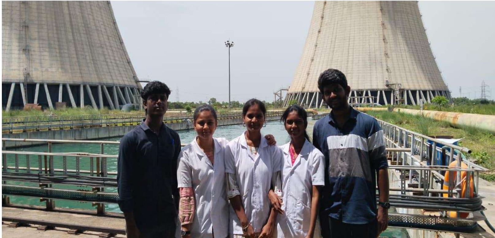
Place: New Neyveli thermal power station (NLC), Neyveli, Cuddalore
